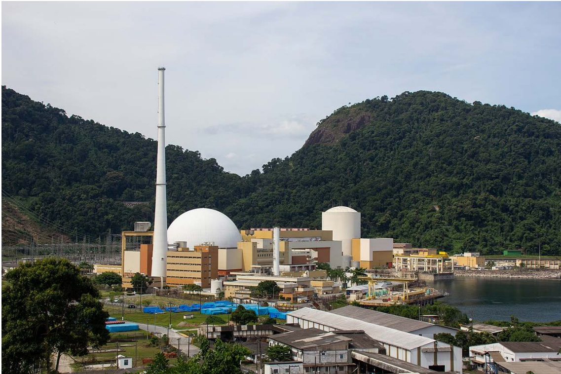
Vista geral da Central Nuclear Almirante Álvaro Alberto, com Angra 1 à direita e Angra 2 à esquerda. https://upload.wikimedia.org/wikipedia/commons/thumb/b/b6/Around_Paraty%2C_Brazil_2018_239.jpg/1280px-Around_Paraty%2C_Brazil_2018_239.jpg
